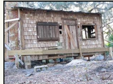
The “levitated” cabin, with foundation and subfloor removed!
