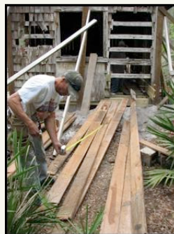
Inspecting and trimming rotten material from sound original floorboards.
