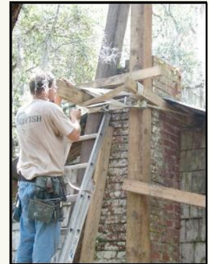
Jeff Penuel secures timber "strong-backs" to chimney prior to "righting."
